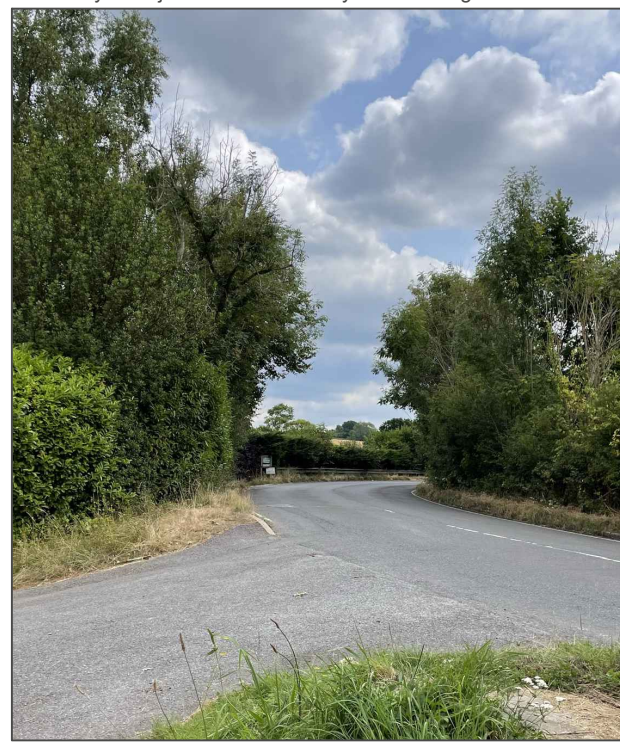
Visibility from junction restricted by dense foliage around bend
