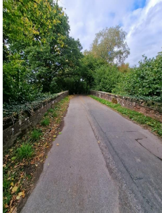
Figure 3-6 Bridge Over Cycle Route
