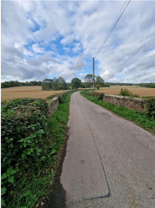
Figure 3-7 Bridge Over River Medway
