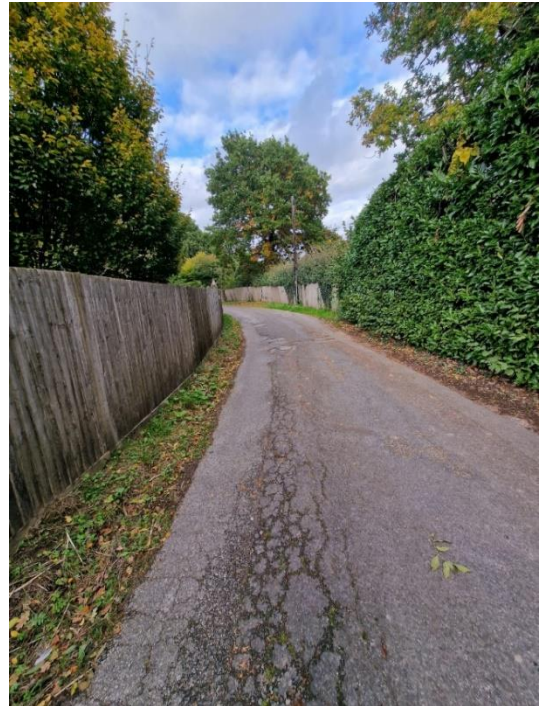
Figure 3-4 Bend in Access Road
