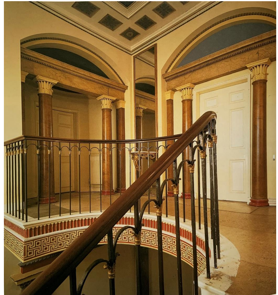
Fig. 12 (above). The upper landing of the main staircase, showing Latrobe's original stair treads and flooring, wrought-iron railing, and his column-screened niches with Tower of the Winds/palmette Coade stone capitals (LHT collection).
